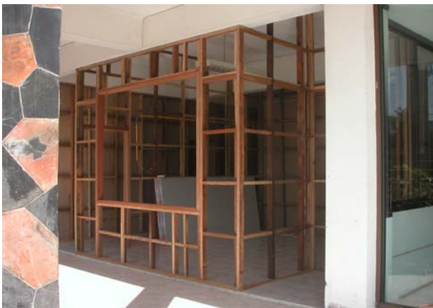
This is one of the classrooms framed up There are 12 classrooms all together
