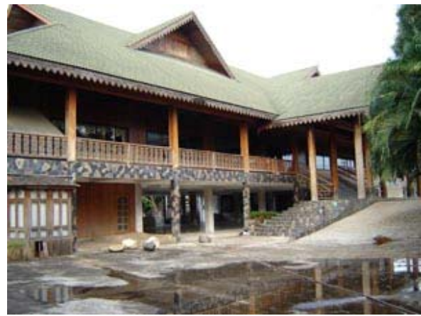
This is the whole building. Pastor's apartment this end, church on top, Family Learning Centre underneath.
