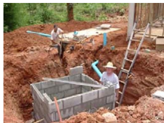
Fraser building a hole within a hole at Mae Chaem
